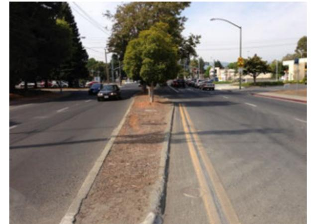
Figure 8: View south towards Central Expressway. Mature trees in median would have to be removed as roadway is to be lowered.
