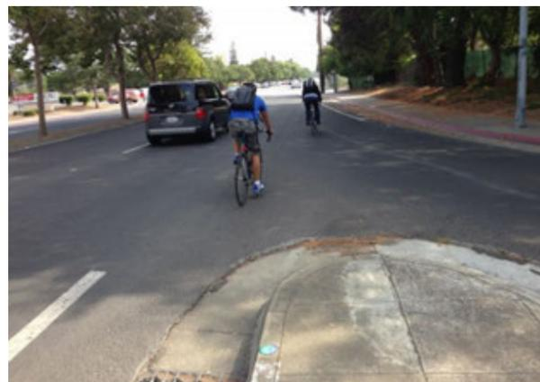
Figure 5: View north on Rengstorff at the north-east corner. Right turn from Central Expressway is a challenge for bicyclists; shallow angle of intersection means that merging motorists must be able to turn their head more than 90 degrees to assess gaps in northbound traffic.
