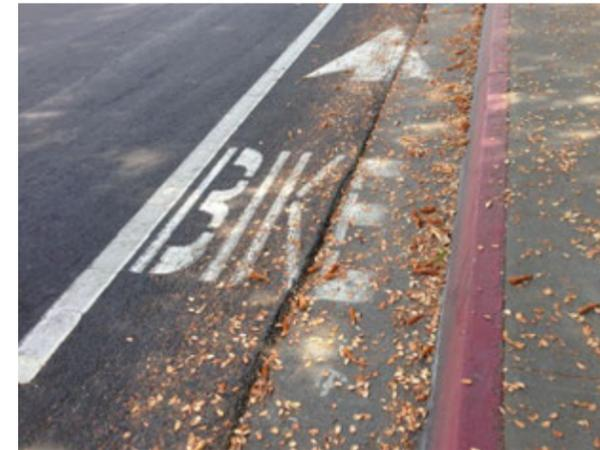
Figure 7: Northbound bike lane is narrow, with a seam between the pavement and gutter pan.
