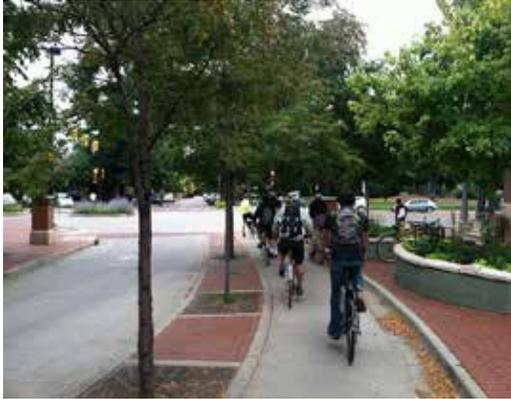
Figure 1-15 A Class IV separated bike lane in Boulder, Colorado
