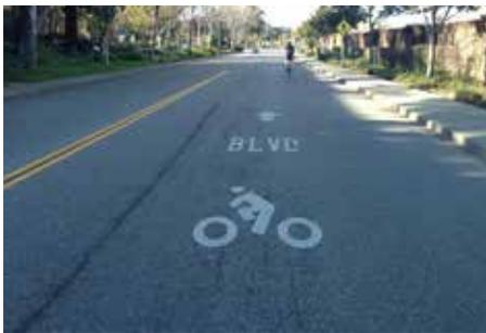
Figure 1-13 Bicycle Boulevard pavement markings on Dale Avenue
